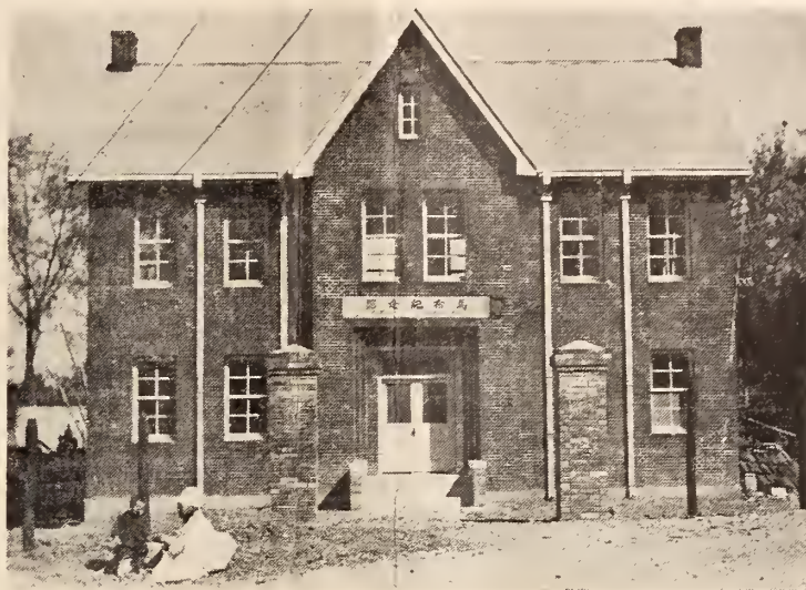
Moffett Memorial Building.
